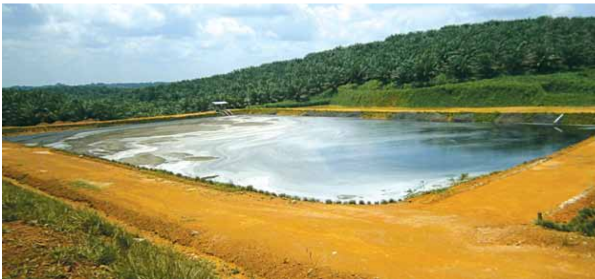
Conventional treatment of POME in open air settlement ponds can be costly to maintain and generate significant GHG emissions. Photo: R. Harjanthi.
